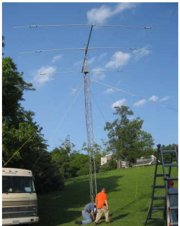
Darian WA4DQ & Ken N4LYO 20 meter tower installation
